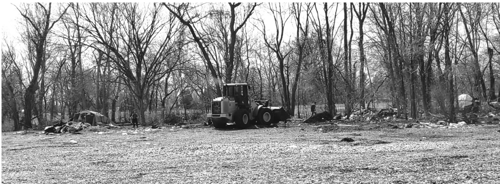
Bulldozer and crews destroying what was left of Mills Camp
